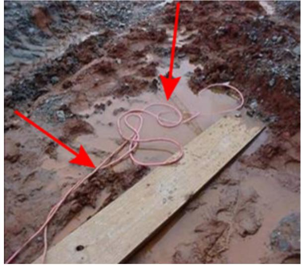
Flexible cord near job trailer should be relocated
